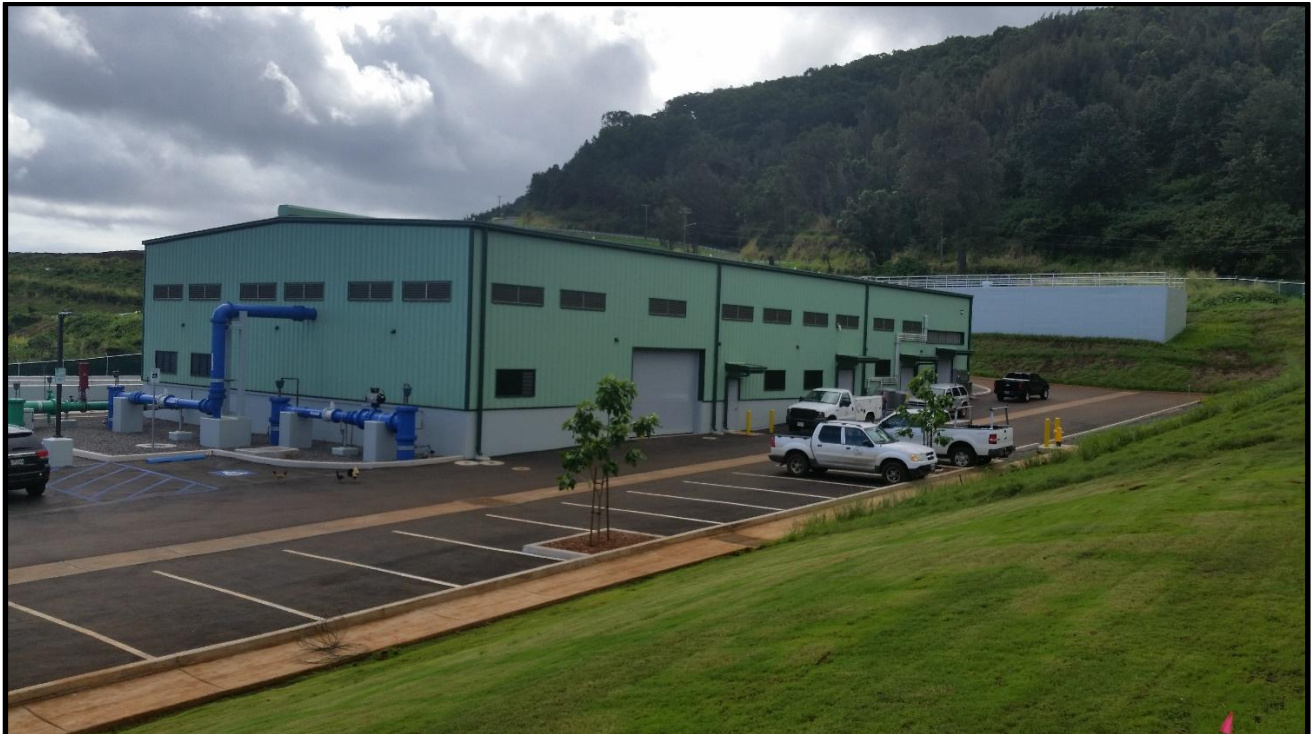
Iao Water Treatment Plant, Wailuku, Maui
