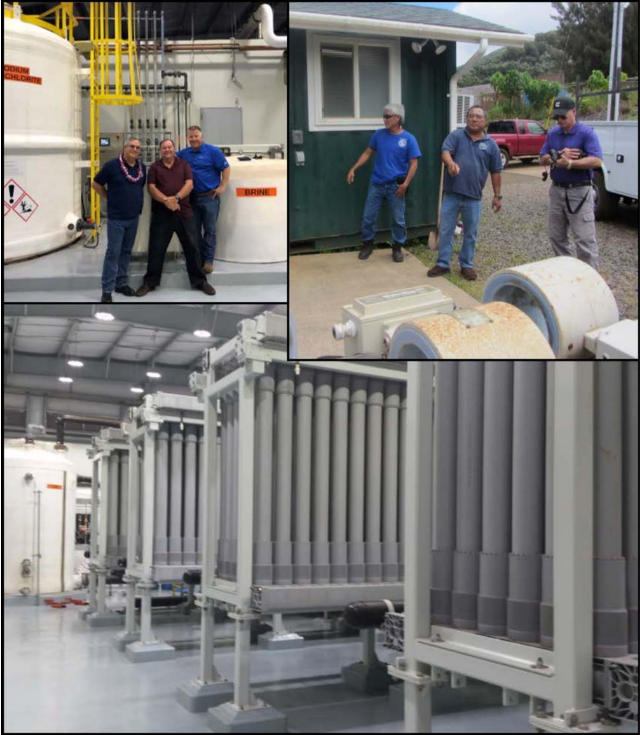
Clockwise from Left: The Blessing/Grand Opening of the new lao WTP. Tony Linder, West District O&M Supervisor David Haddock and O.S.G. contractor Rob Crow from Aqueous Vets; Lloyd Shiraki, Marvin Ignacio and Tom Ochwat working the decommission of the old lao Water Treatment Plant; The membrane filtration system of the new lao Water Treatment Facility.
